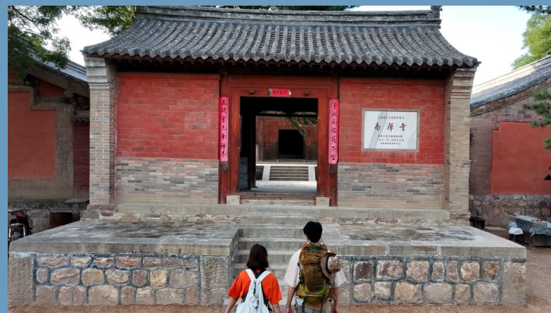
Exterior of Nanchan Temple in Shanxi Province
